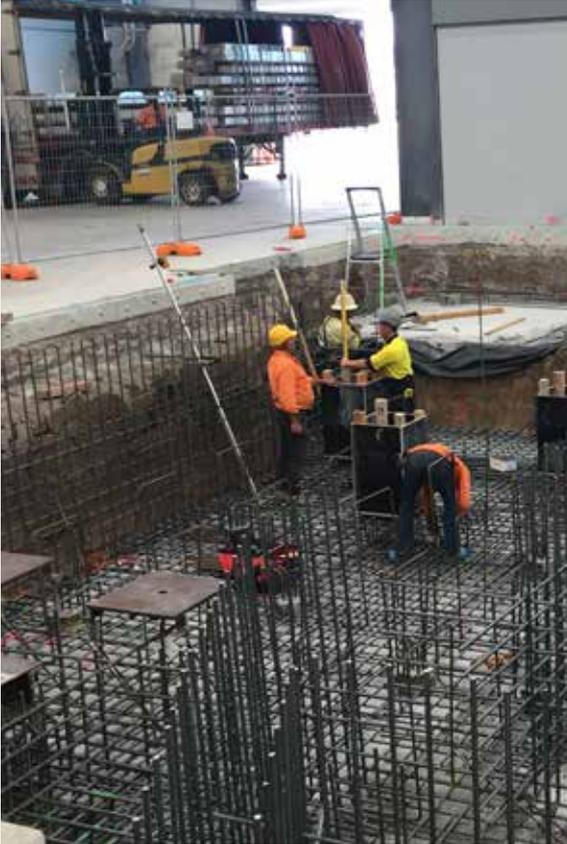
The bearing capacity of the concrete foundation directly determines the rigidity of the overall mechanical structure and is integral to the processing precision of heavy machinery tools.
