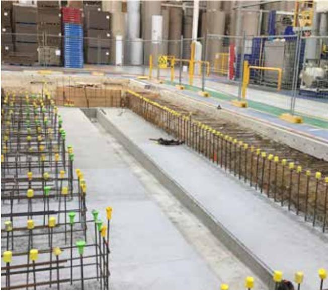
**Correct load bearing capacity and structural rigidity** is critical to maximise machinery performance and to minimise machinery deterioration and/or vibrational impacts to surrounding work environments. We are experts in managing the professional steel and formwork required to achieve necessary load bearing capacity and structural rigidity of machinery foundations.
